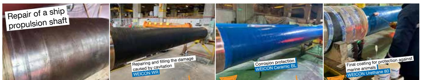
Repair of a ship propulsion shaft
