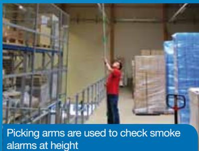
Picking arms are used to check smoke alarms at height
