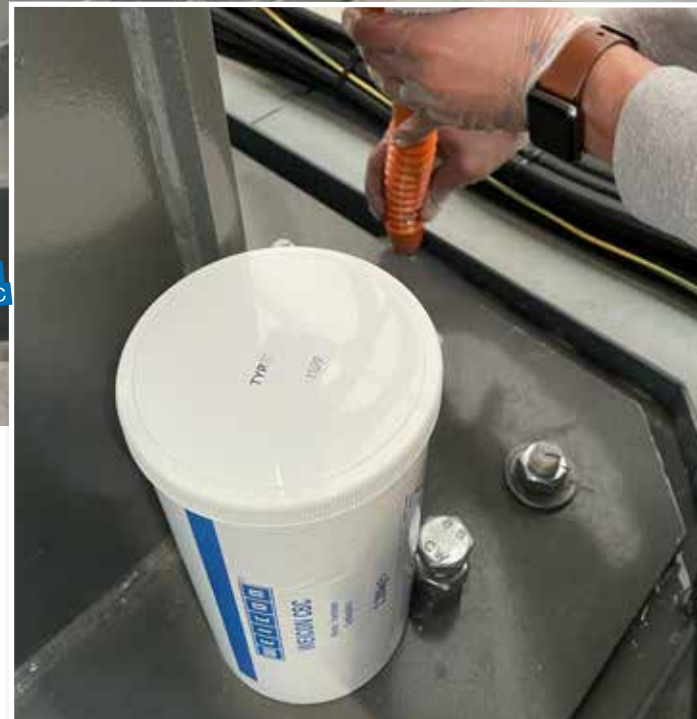
Lining a machine foot WEICON CBC
