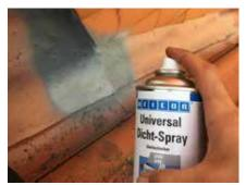
Right next to the chimney, there is a skylight window. In order to seal it, Dennis used Allround Sealing Spray again - the black one this time.
