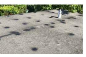
nails became rusty due to weather conditions and formed fine cracks in the roofing felt. For protecting the roof from moisture, Philipp sealed all nails with Allround Sealing Spray Black.
