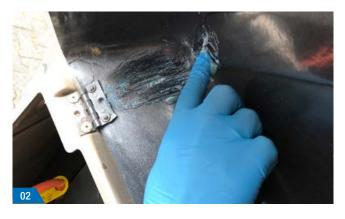
**Step 2:** Apply the adhesive evenly to the inside of the gas locker box over and around the crack.
