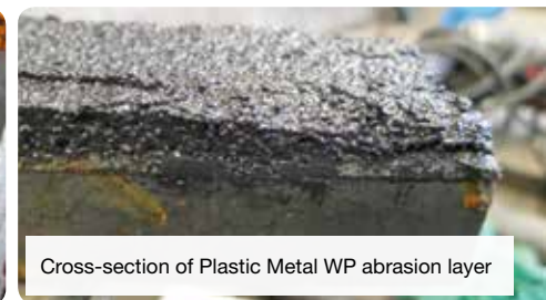
WP - Sag mill chute liner repair & wear protection
