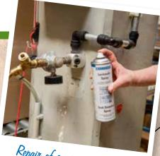
Repair of compressed air lines
