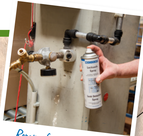
Repair of compressed air lines 💰 1,151 € ⚡ 7,498 kWh
