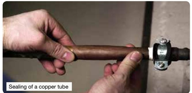
Sealing of a copper tube
